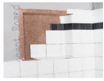
thicker bed of bonding material at the front or rear of horizontal plane as necessary. Do not adjust slope to angle backward toward rear of unit.
