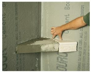
Tile and grout the top and front face of the Better-Bench® as desired.
