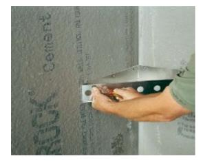
Remove screws and inject a small amount of adhesive caulk in each mounting hole. Reposition Better-Bench®, insert fastener or wood screw and tighten completely using a hand screwdriver.
