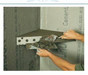
Place a continuous bead of adhesive caulk along top edge of the Better-Bench® at wall surface. Apply stiff mortar to completely fill bench unit, allowing for surface drainage by building mortar up in back corner and screed even with upper front lip of unit. Pack mortar tightly, allowing the mortar to press through the front holes. Fill in any voids in front channel and screed mortar flush with upper and lower lip of channel.
